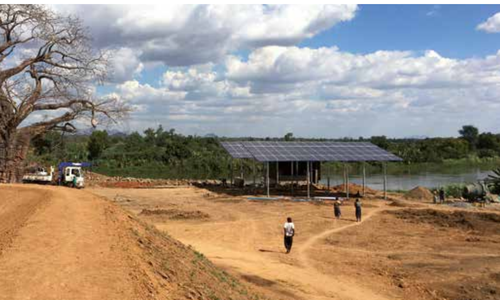
Solar powered irrigation projects
