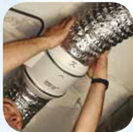
Acoplar as condutas
